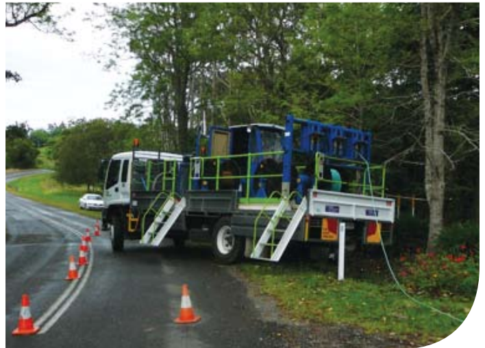
The new winch in action
